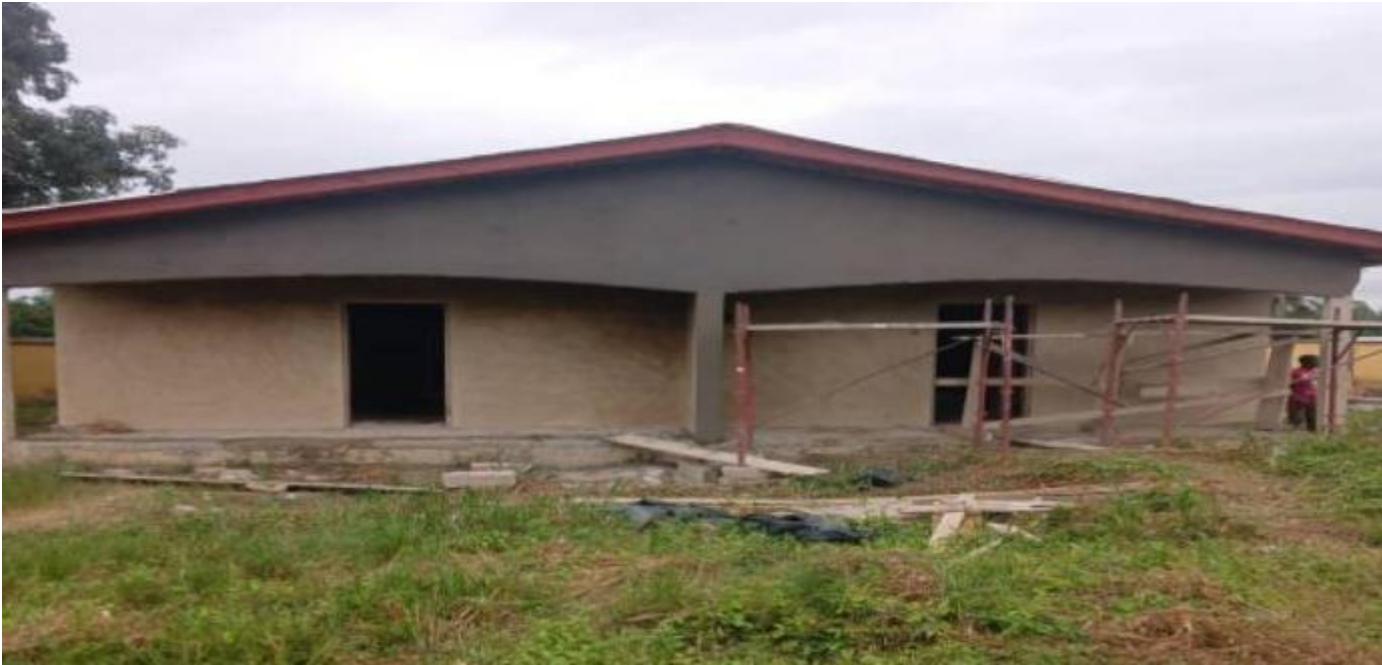
Constructed 16-Seater W/C with 4 Bathrooms at New Abirem
